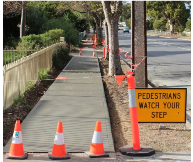
Kerb and Footpath works
