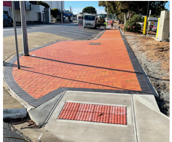
Footpath paving King St
