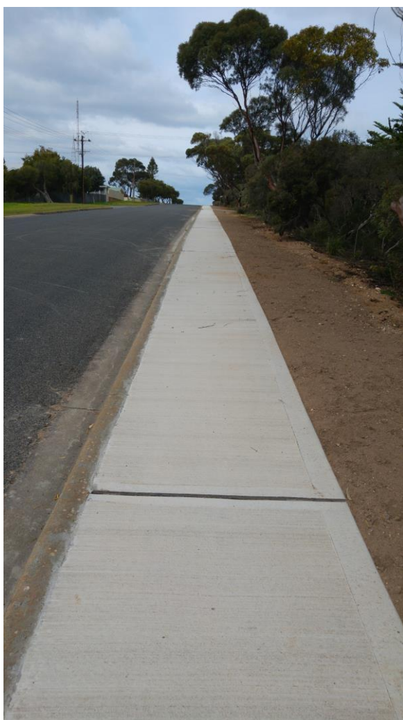
Photo 3 – Newly laid insitu concrete footpath looking South East along Cardiff Road
