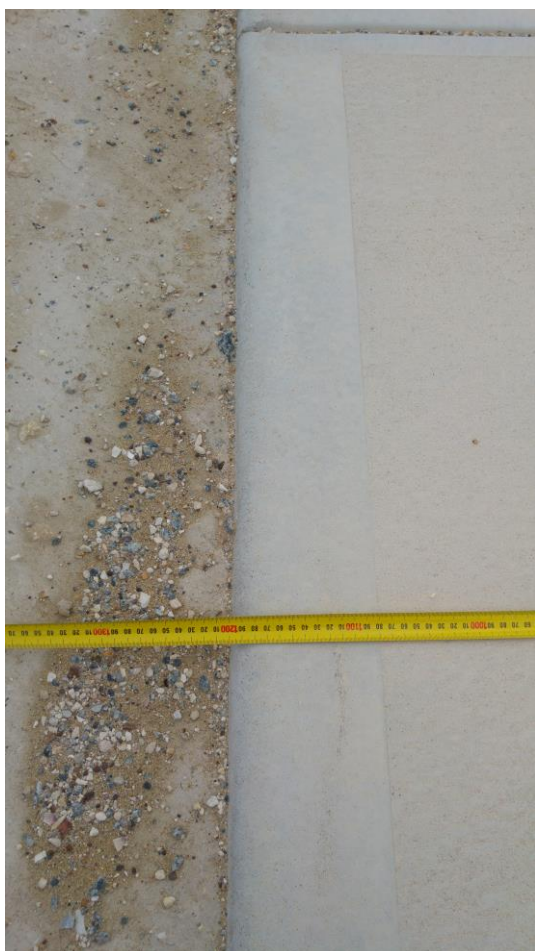
Photo 8: Measure of installed 1.2m wide concrete footpath at Delamere Drive
