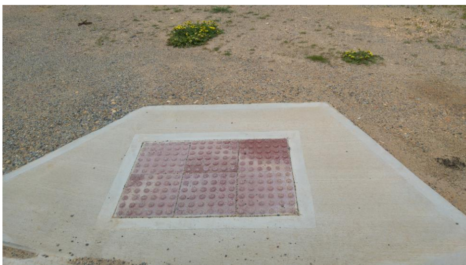
Photo 9: Pram ramp installed with kerb in preparation for construction of insitu concrete footpath by developer at Delamere Drive
