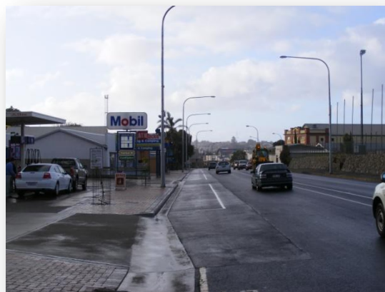
Figure 29 PLEC Underground powerlines and street scaping
