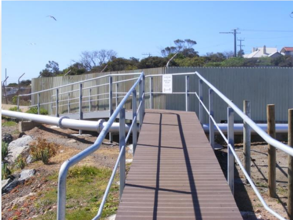
Figure 30 Parnkalla Trail ramp over pipework
