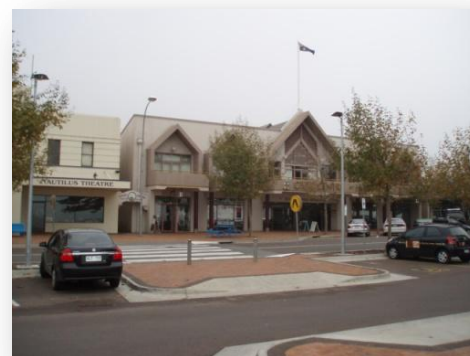
Figure 17 Civic Centre from Tasman Tce
