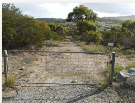
Figure 38 Upgraded Fire Track Access
