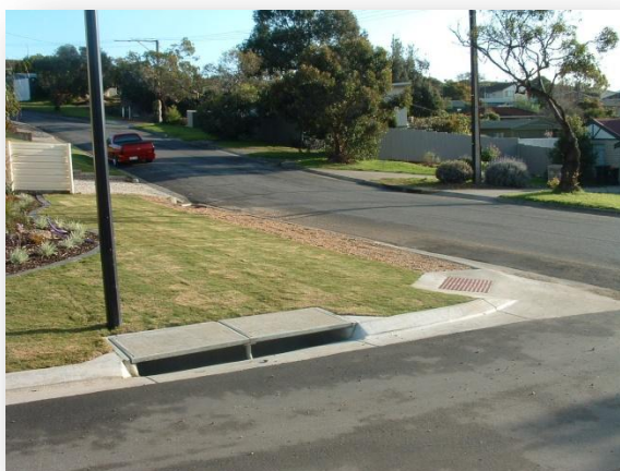
Figure 28 New Kerb, Guttering and Drainage
