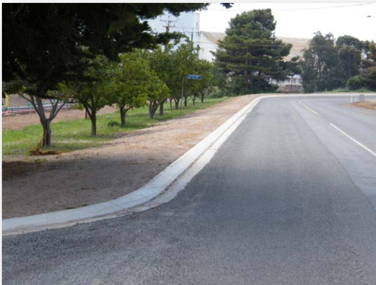
Figure 18 Stevenson Street road works
