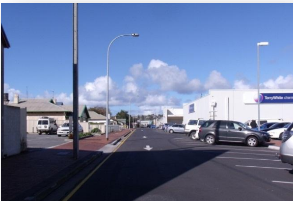
Photo 13 Washington Street PLEC & One way Upgrade
